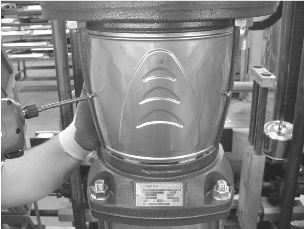
Removal of coupling guard
